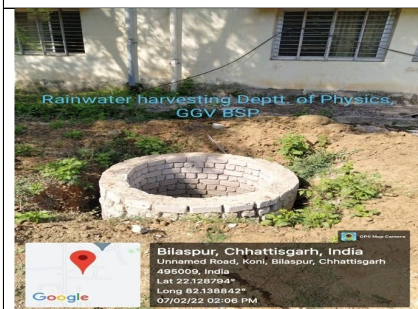
Rain Water Harvesting @ Physics Department
