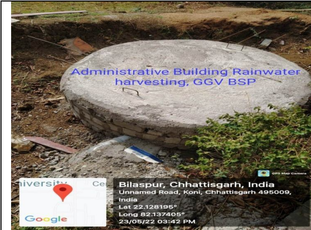
Rain Water Harvesting @ Administrative building
